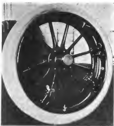
HOW THE STEPNEY WHEEL IS FITTED.
